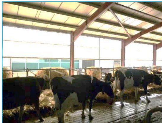
Figure 1 : Surfaces ventilantes modulables (Source : GDS12)
